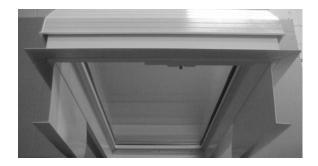
7- The trim kit sides are premanufactured for 6" thick roof panels. The corners are notched to allow for the vinyl welded joint in all four corners of the skylight curb. The trim kit sides are scored for ease of cutting down to be used for 3" or 4" thick roof panels. If cutting is required to the trim kit sides they will need to be notched at the ends of each panel. Use manufacturer's notch as template.
